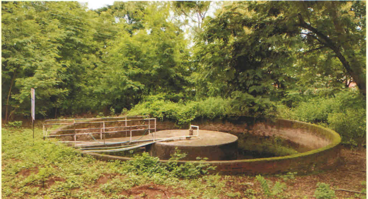
Rain Water Collection Well at Shivaji Arts & Science College, Chikhali
